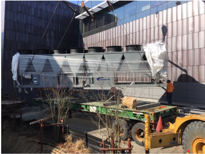
Cooling system is lifted by a crane, rotated, and lowered onto a platform along the south side of the Kashevaroff Building.
